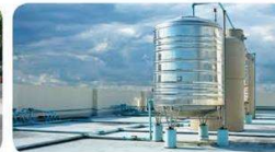
Water Tower Supply
